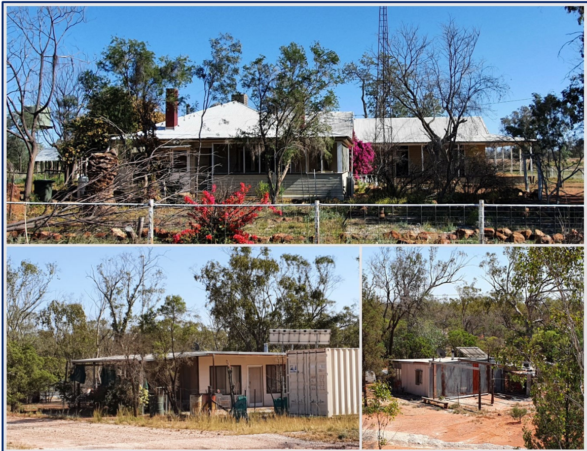
Figure 13 – Residences on the Reserve Clockwise from Top – Wandella Homestead; Residential Mineral Claims at Glengarry; Residential Mineral Claims at Grawin.
