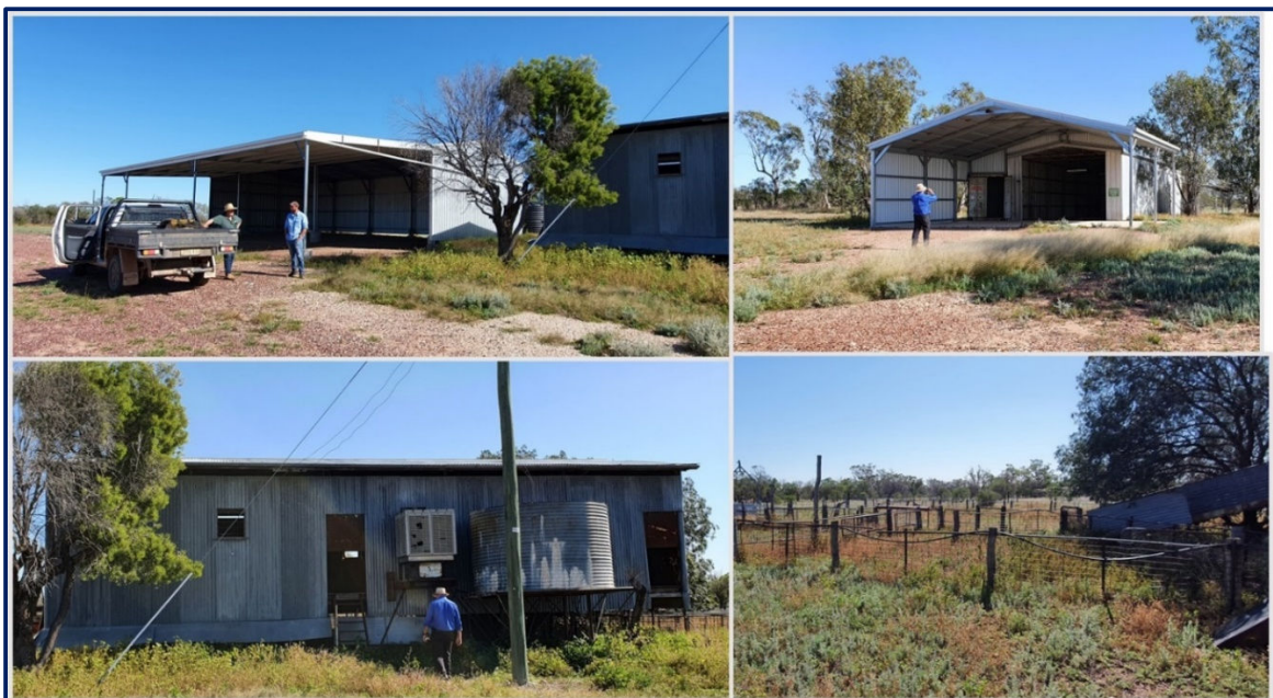
Figure 27 – Infrastructure at Rexeen.
