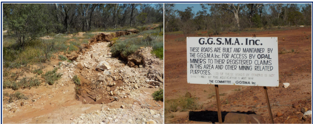
Figure 41 – Track and Road Maintenance Roads works are inadequate across the Reserve.
