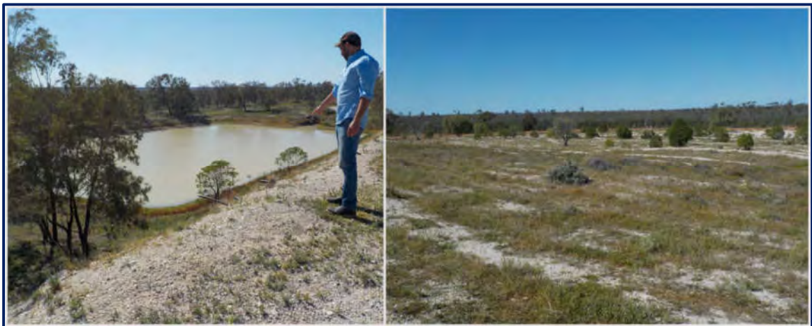
Figure 36 – Rehabilitation Dam used as water supply for opal mining wet puddling/agitation (left); Rehabilitation of disturbed site uses contour ripping and reseeding.
