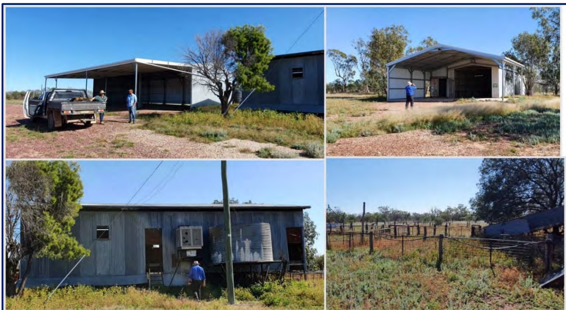
Figure 27 – Infrastructure at Rexeen.
