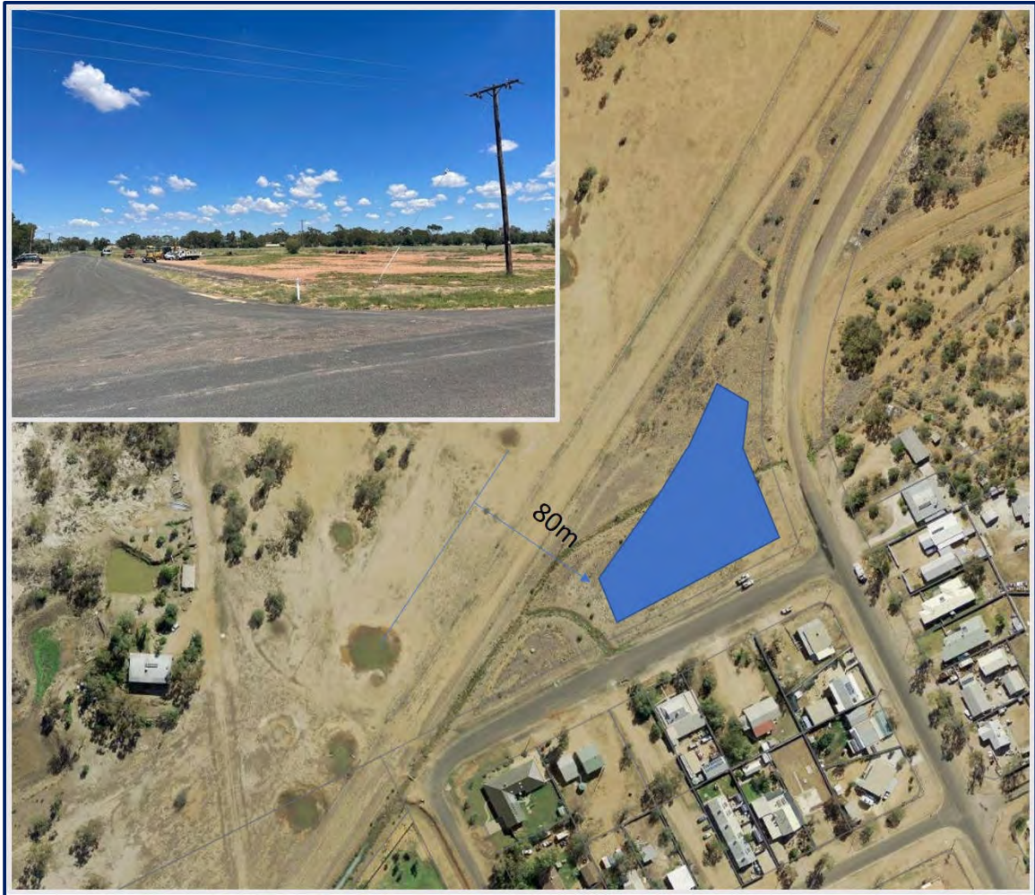
Figure 53 – Possible Tourism and Recreation Sites Possible Site for Hotel lease – Cnr of Gem St and Kopi St.
