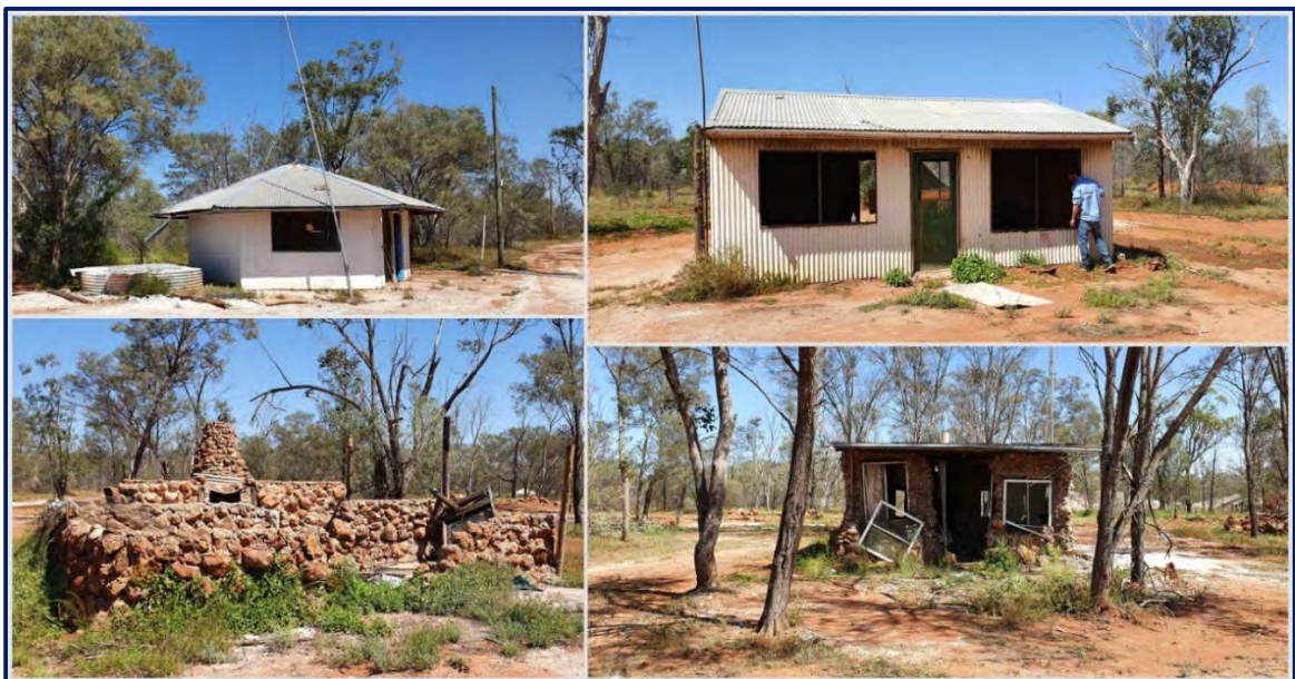
Figure 28 – Infrastructure - Garule-Wali Reserve.
